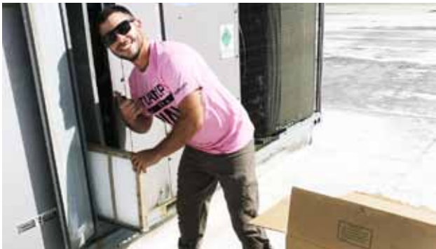
Blake Eads of Berger Mechanical installing a Glasfloss filter in a commercial unit
