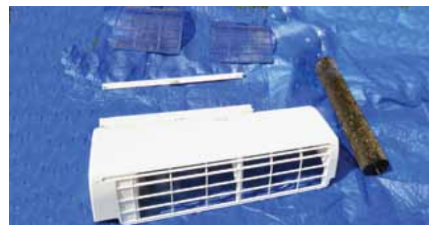
The ductless mini-split parts were all cleaned and dried off in the sun
