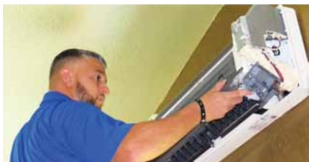
David Diaz of CoolAir disassembles the mini-split unit to clean the dirty blower wheel, evaporator coil, and other removable parts
