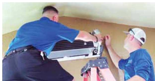
David Diaz and Steven Krzyzanowski of CoolAir reinstalled all the cleaned mini-split parts and prepared to install the Mini UV LED
