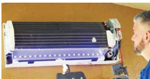
The Fresh-Aire Mini UV LED disinfects the mini-split blower (highly prone to mold growth) and improves indoor air quality
