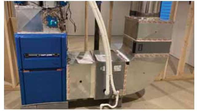
HVAC System indoor
