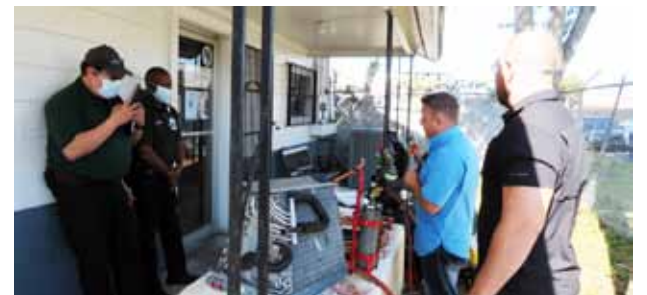
Ray Diaz and Fredrick Cintron of Advent Health with Chris Craft and Andres Ponce of Target Sales repairing an aluminum coil
