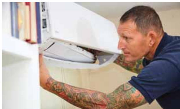
B&B Cool Air technician hangs a wall-mount evaporator on the living room wall
