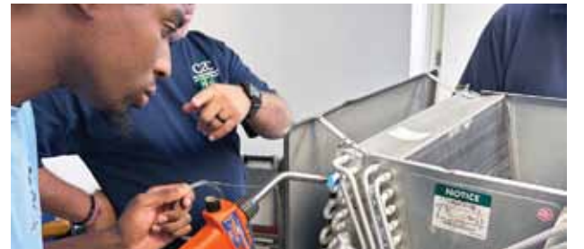
Everyone who attended the training successfully repaired a leak in an aluminum coil using the appropriate torch and alloy.
