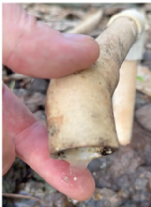
HVAC condensate completely laden with Zoogloea
