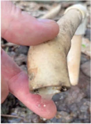
HVAC condensate completely laden with Zoogloea
