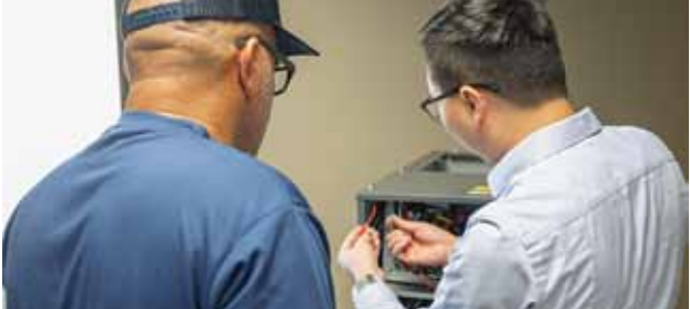
Keith Lau of TGM shows technician proper installation wiring of TGM interior air handler components
